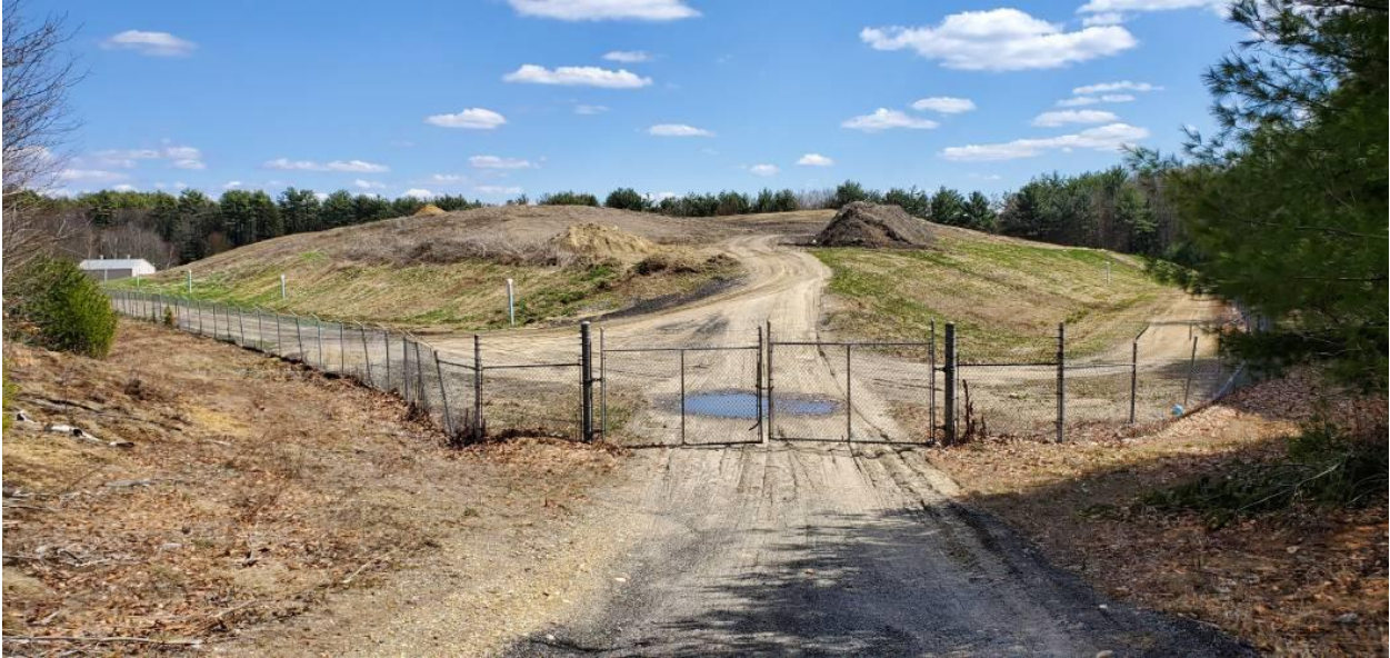
The proposed Gardner sludge landfill gets very close to the Otter River, which is a major tributary of the Millers River. Athol Daily News file
